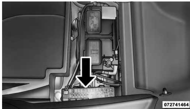
Rear Power Distribution Center
